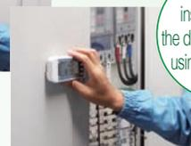
It can be installed inside the distribution board using the magnet.
